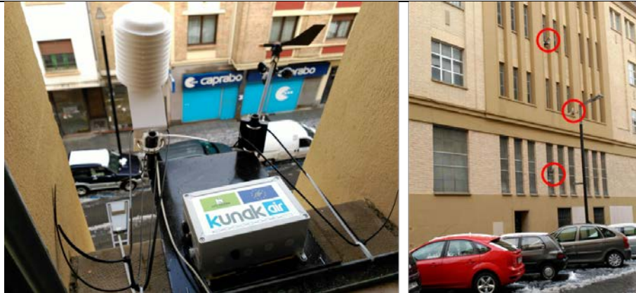
Figure B4.7. Measurement of atmospheric pollutant concentration and meteorological parameters at different heights in a street canyon in Pamplona.
