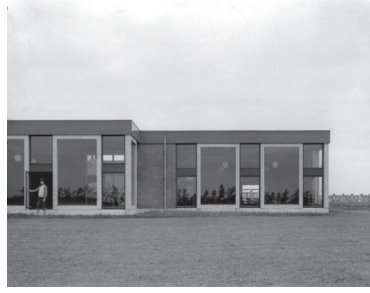
Fig. 1. Aldo van Eyck, Daniel van Ginkel, Schools in Nagele (1954-1956). Stepped exterior of the class rooms. Source: Das Werk: Architektur und Kunst , n° 45 (1958).
