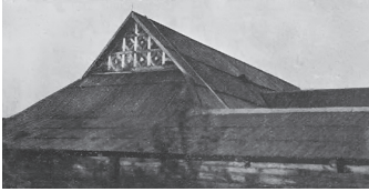
Fig. 6. Gable decoration of a Hutsul house, 1933.
