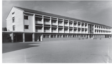
Fig. 9. Rear façade of the building and detail of a window of the classrooms of Liceu Rainha Dona Leonor.
