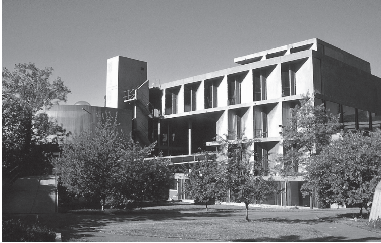
Fig. 8. Carpenter Center, rear view, west façade, with walls and angled brise-soleil in smooth 'béton brut' for protection from direct rays of sun. The ramp descends towards Prescott Street.
