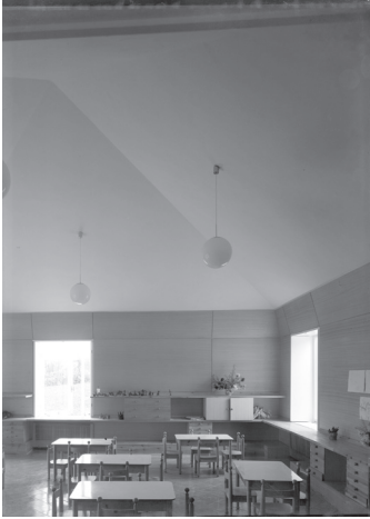
Fig. 6. One of the classrooms in Gubbio. The boiserie marks the construction lines that make up windows and doors. Every piece of furniture raises up to 50 cm to coincide with the windowsills and to be reachable by children. The same height can be appreciated in the stone base in the outside elevations (1960). Photo by Giorgio Casali. Università Iuav di Venezia. Archivio Progetti, fondo Giorgio Casali.
